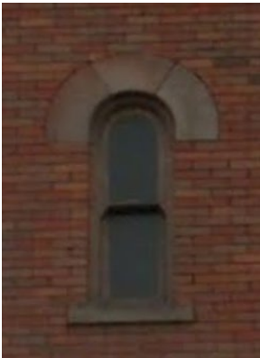
Third-floor accent arches
